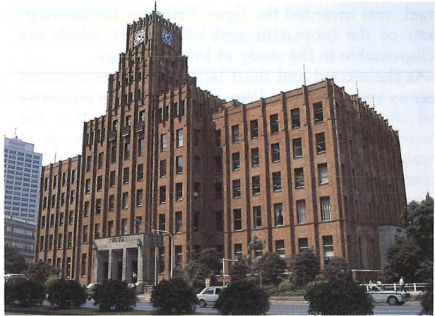
Shisei Kaikan, where the Main Office of the Foundation is located.
